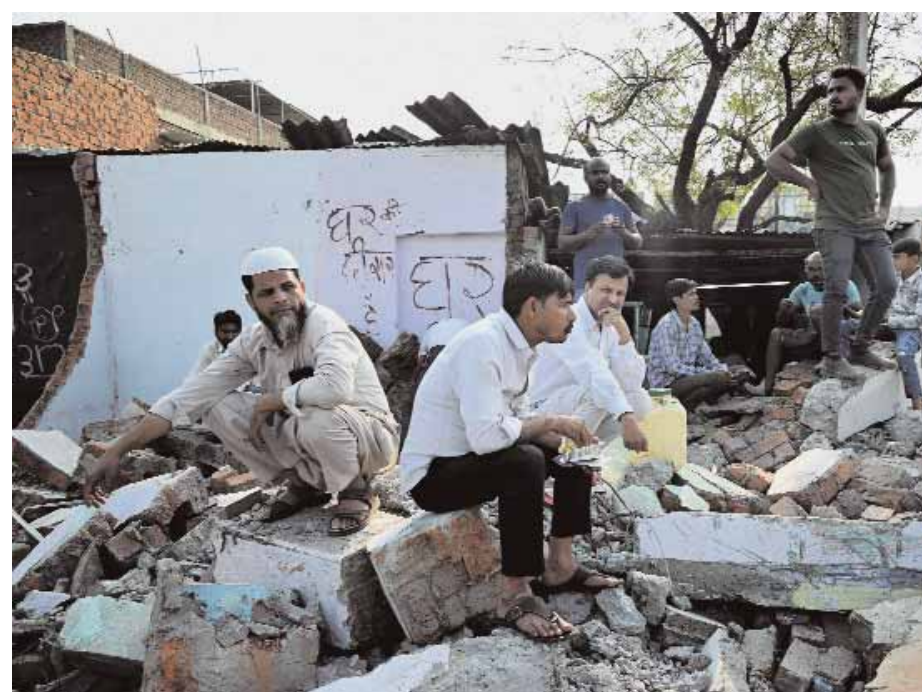
BMC employees demolished houses and shops to clear the venue following the order of the district administration for the expansion of railway track at Motinagar, old Subhash Nagar locality in Bhopal on Sunday. Pioneer photo
